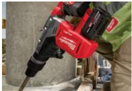
Drilling multiple back-to-back holes in concrete
